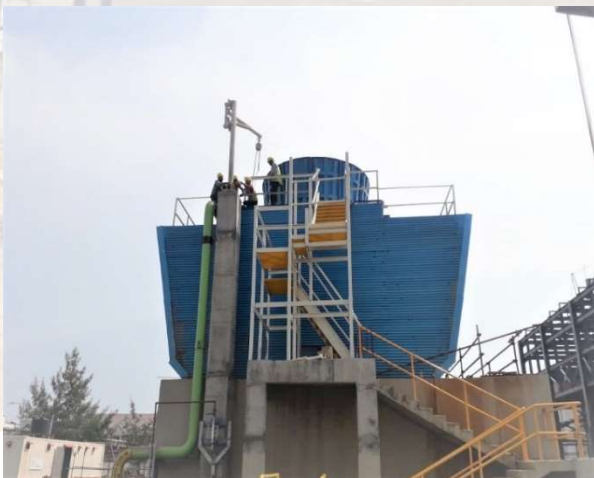
DAVIT ARM AND DOUBLEDECK STAIRCASE
